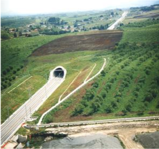
The Gelsi tunnel
